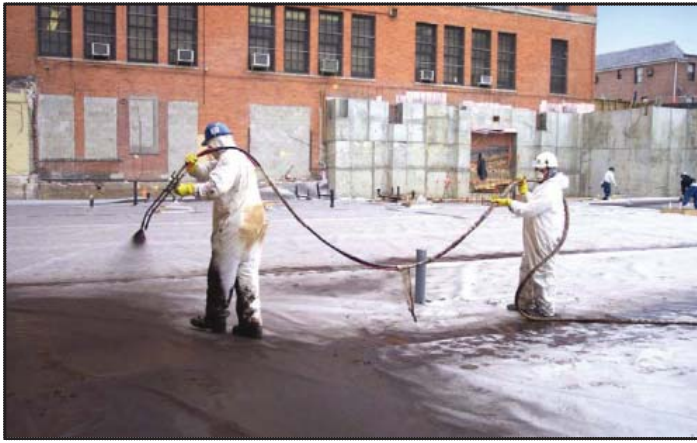
EAI employees dressed appropriately for a jobsite installing Liquid Boot®.
